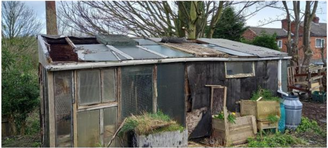
General View of Shed to be replaced
