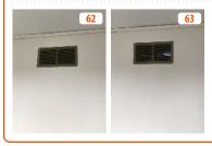
Seal breach in the fire compartment to provide a minimum of 30 minutes fire resistant protection.
